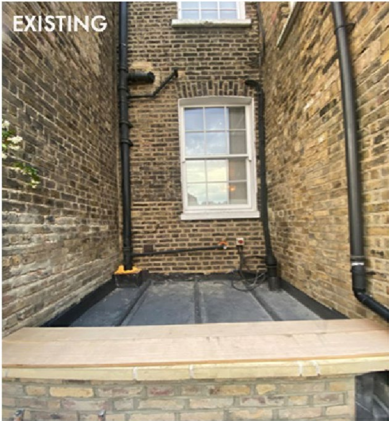
Photograph of first floor flat roof
